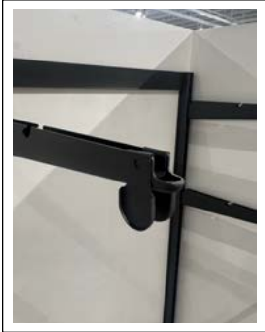
Install Light Clips on inside of Brackets.
